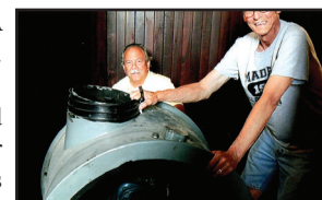
L-R Kevin Finazzo and Jim Fesler Removing the old blower system
