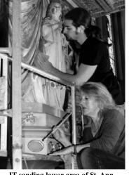
JT sanding lower area of St. Ann while Michele brushing on chemical to perform controlled paint removal
