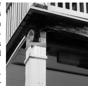
Rotting support timbers replaced with treated wood.
