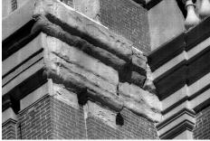
new element of the work, A striking difference: Unrestored dissolved stone surfaces between completed restored areas.
