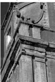
Typical deterioration of stone on corners and horizontal surfaces.
